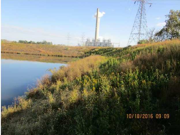
Picture 7 – Clear Water Pond, overgrown vegetation on inboard slope
