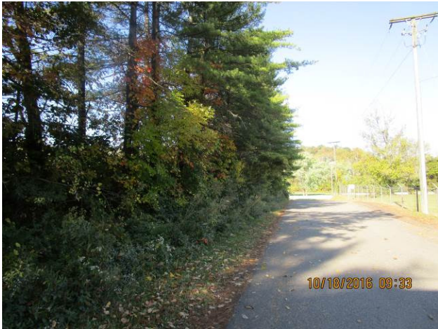
Picture 9 – Boiler Slag Pond, trees on outboard slope
