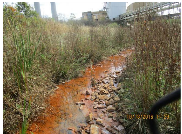
Picture 21 – South Fly Ash Pond, seepage area beyond south dike.
