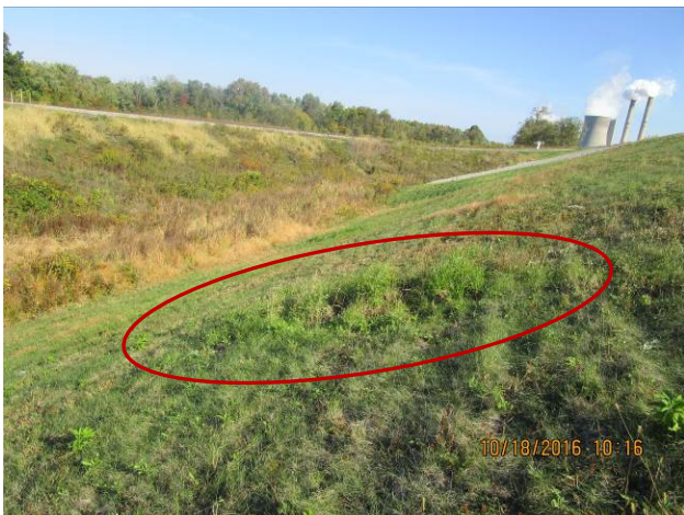
Picture 14 – South Fly Ash Pond, west dike wet area along outboard slope
