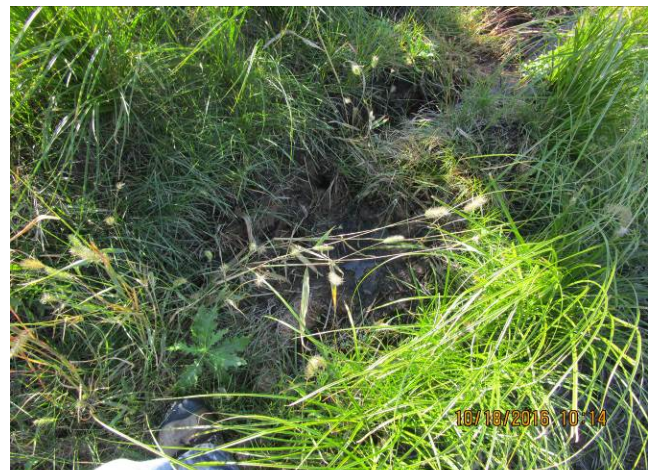
Picture 15 – South Fly Ash Pond, wet area along outboard dike
