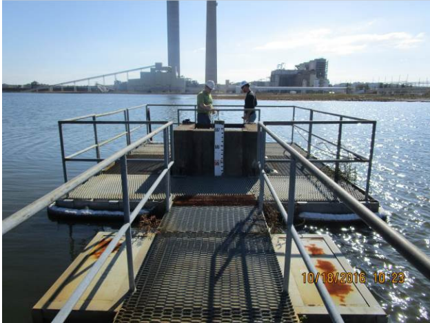
Picture 10 – South Fly Ash Pond, General View of Outlet structure
