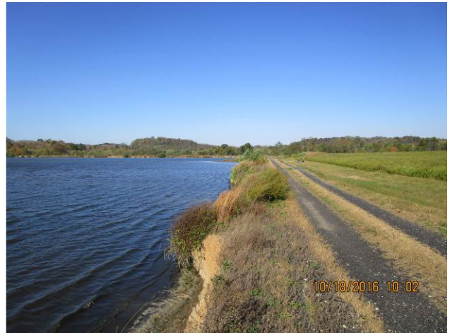
Picture 13 – South Fly Ash Pond, wave erosion at north dike
