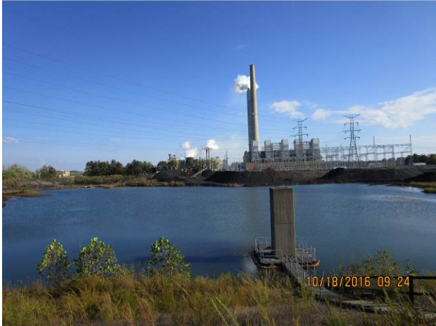
Picture 1 – Boiler Slag Pond, Overall view
